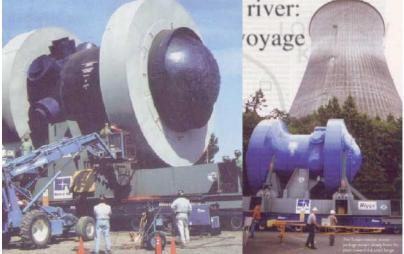
Figure 2-4 Loading of the RPV onto a Barge adjacent to the NPP
