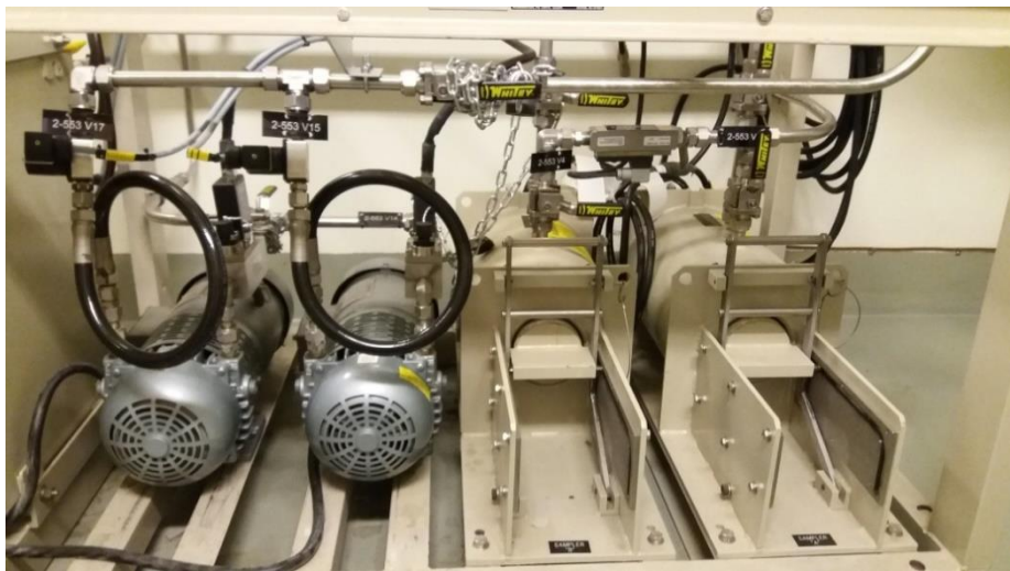
Figure 3-4. Aerosol sampling at B2 in the activity monitoring system. The pumps in secondary loops and cartridge holder cells are shown. The system at B1 has a similar design.
