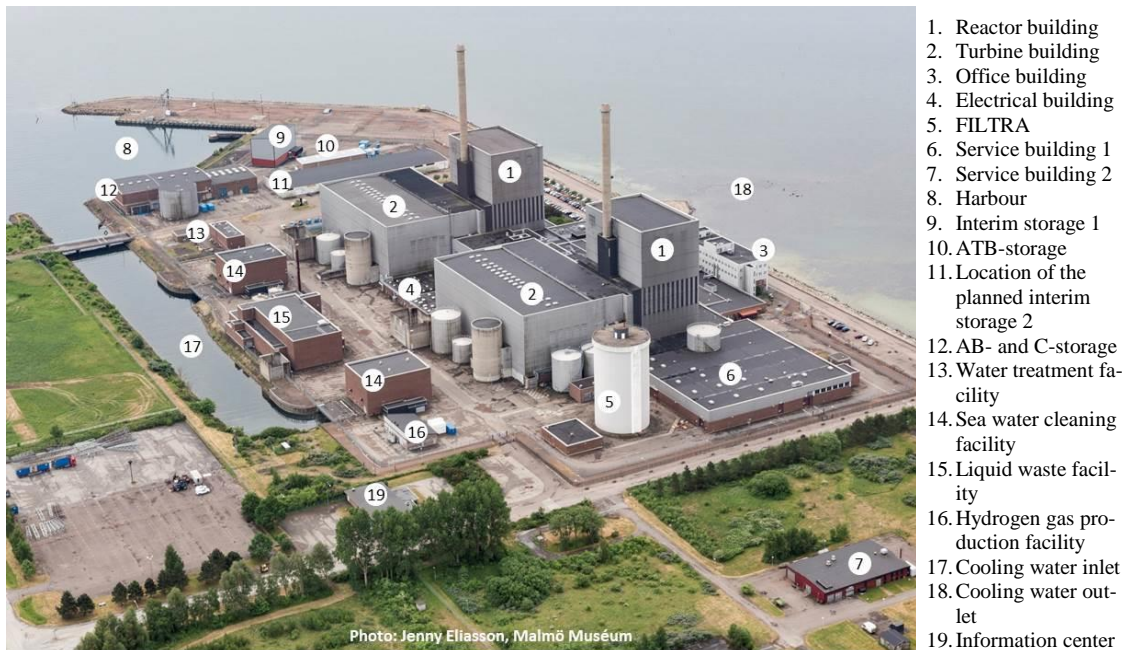
Figure 2-1. Barsebäck nuclear power plant. Note that no. 11, pointing out location of the planned interim storage 2, actually shows the goods reception building that will be demolished in favour of interim storage 2.
