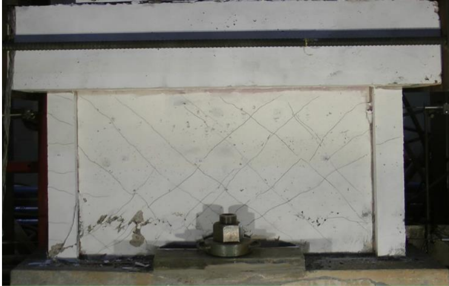
Figure 2-29 Failure (cracks width not measured) of Reg B [15].
