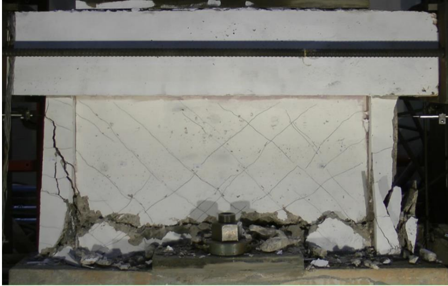
Figure 2-31 Failure (cracks width not measured) of Reg B [15].
