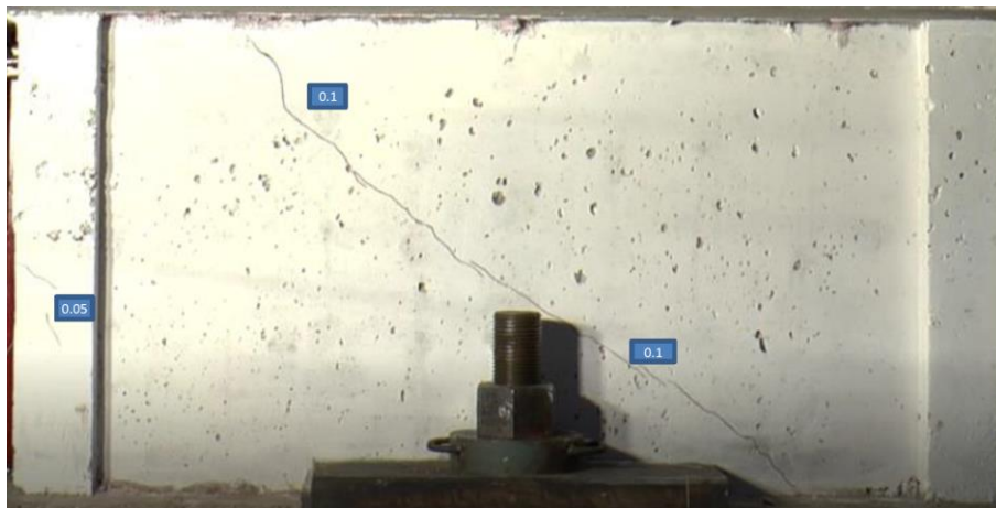
Figure 2-45 First crack at a load of 945 kN and a displacement of 0.8 mm of ASR B1 shear wall [15].
