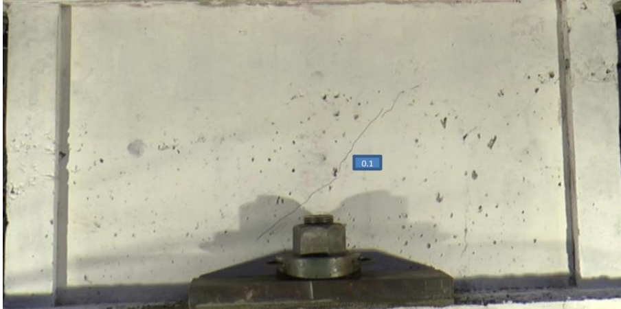
Figure 2-53 First crack at a load of 568 kN and a displacement of 0.4 mm of ASR B2 shear wall [15].
