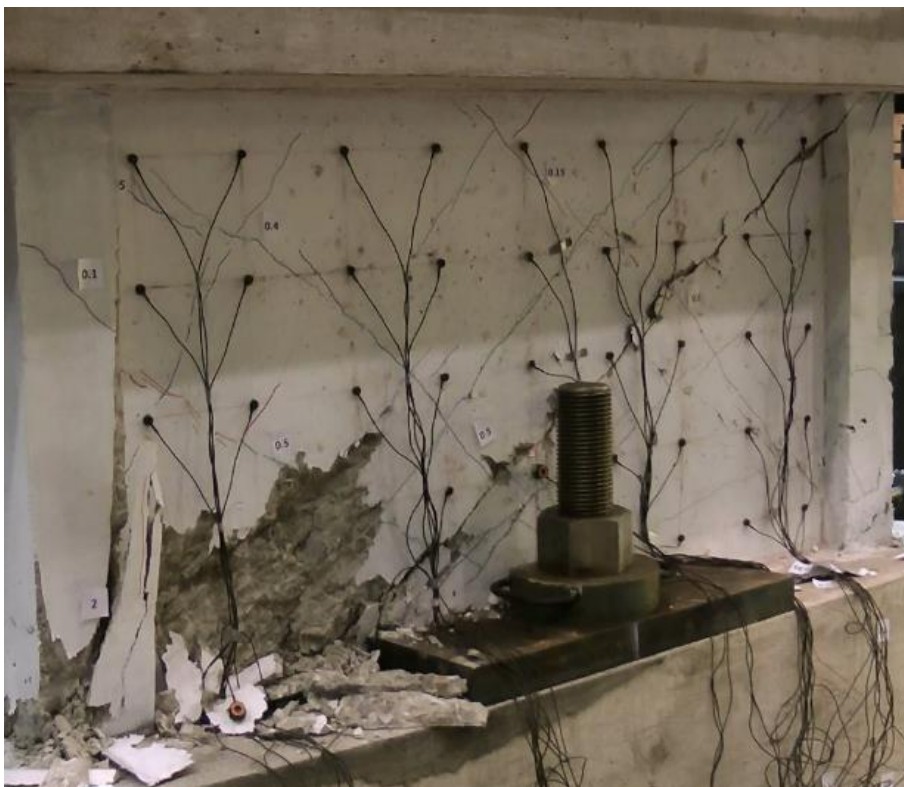
Figure 2-20 Failure (cracks width not measured) [15].
