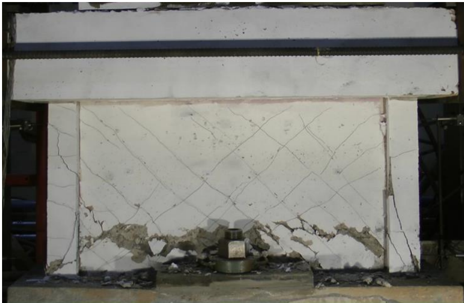
Figure 2-30 Failure (cracks width not measured) of Reg B [15].
