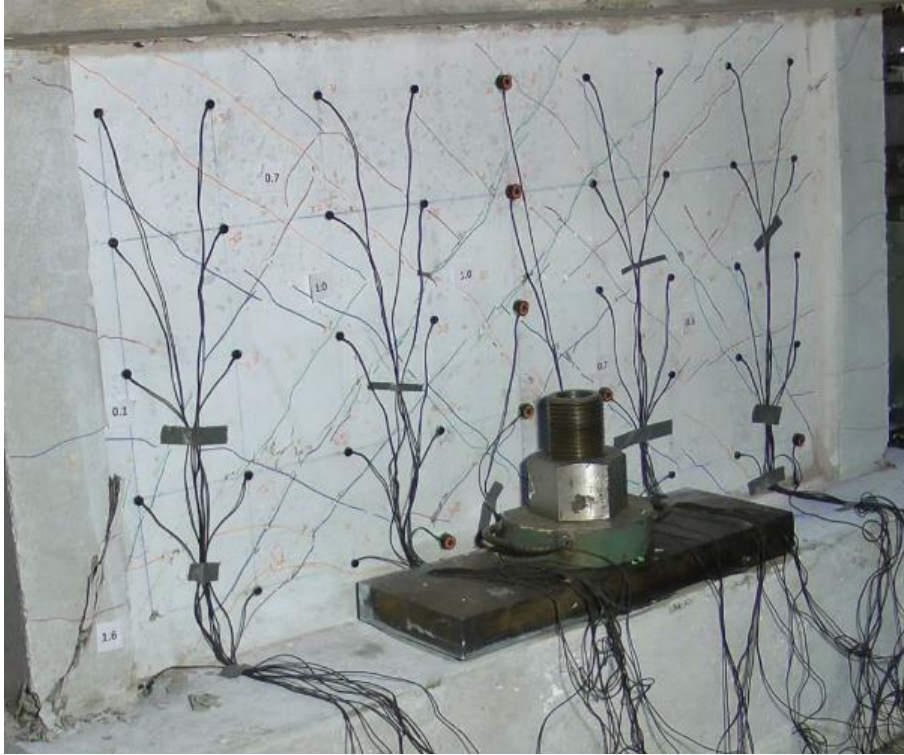
Figure 2-38 Failure (cracks width not measured) of ASR A1 [15].
