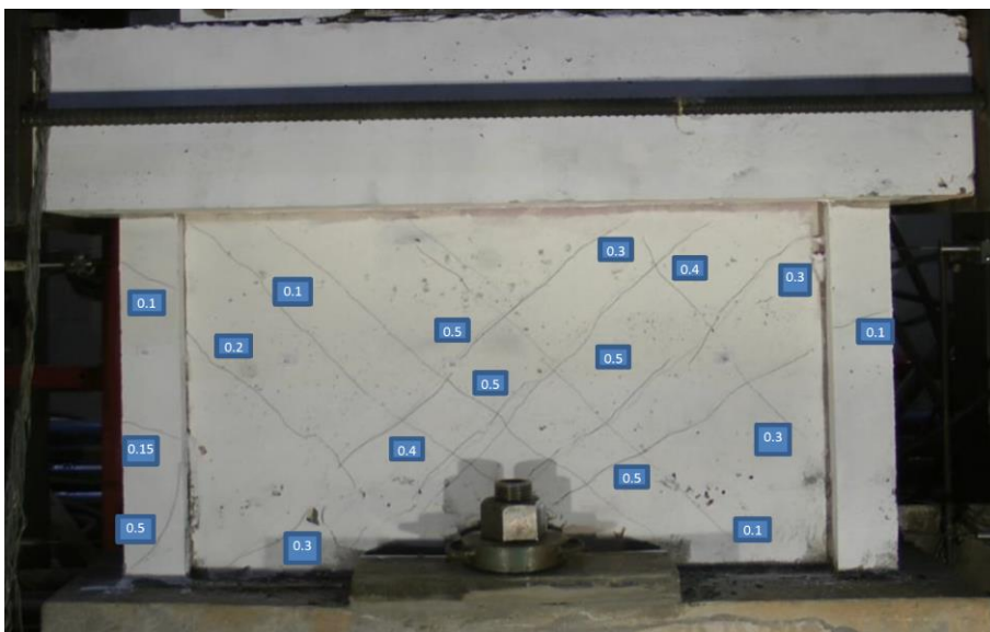
Figure 2-28 Peak load 1181 kN and a displacement of 5 mm of Reg B shear wall [15].
